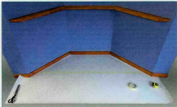
Cut the wall paper or lining paper to the exact shape of your bay...
