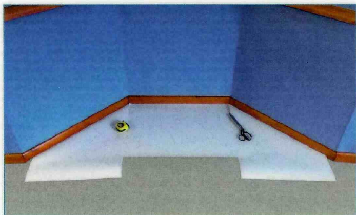
Fold the paper into the corners of the wall/skirting...
