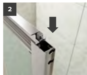
2 Slot the horizontal profile and screws into upright using guide channel until flush
